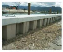
Tidewall sheets were used to construct a secure, permanent wall around a new high-end marina in Tauranga, New Zealand. Tidewall was chosen for its combination of aesthetics, corrosion resistance, and low cost. Precast concrete sections were placed atop the wall, and the final result is a beautiful wall that will last for decades.
