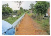
Tidewall was installed as a flood wall on several canals prone to flooding. The earthen dikes would erode and fail, allowing the flood waters to breach the dike. The Tidewall sheets were driven into the center of the dikes, with the wall projecting above the top of the dike to a specified height, providing a permanent solution to the flooding problems.
