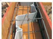
Tidewall was installed as a flood wall surrounding a valuable commercial installation. Thailand experienced a major flood in 2011, resulting in a need for cost-effective floodwalls throughout populated areas. Tidewall was an ideal solution; a 2 meter high wall finished with a steel reinforced concrete cap.
