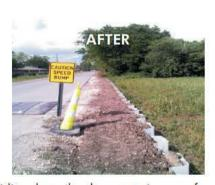
Due to the extreme slope of the land, this road in Lafourche Parish in Louisiana was cracking and sliding down the slope, causing unsafe conditions and resulting in ongoing repair expenses. The problem was corrected using Tidewall TW75 in 3 meter long sheets, with approximately 2/3 meter of exposed height. This brought the shoulder of the road closer to the elevation of the road itself, relieving the stress on the asphalt and allowing permanent repairs to be made.
